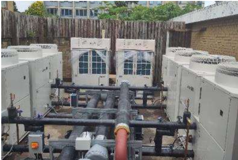
Haldane Building, air source heat pump
